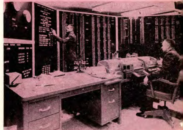
NORAD Space Defense Center. Tracking information from several sources is computer processed and displayed on status boards in Center.
